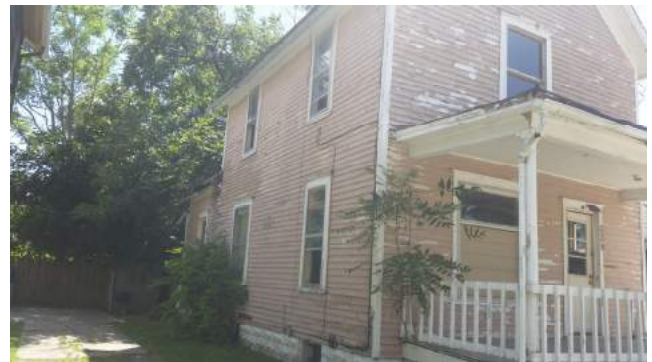
Side #2 of house/property
