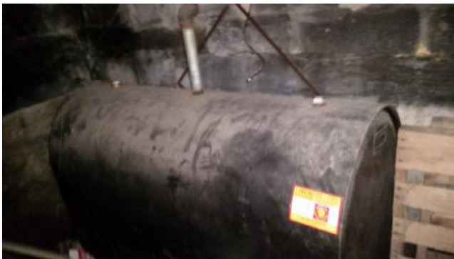
Above Ground Storage Tank: Appears Empty, Room 13
