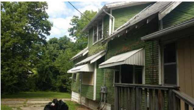
Back of house/property
