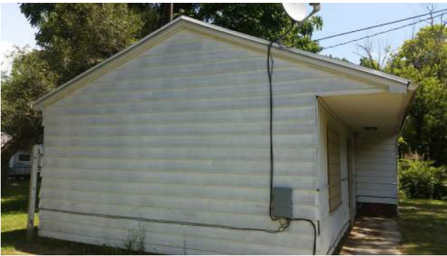
Back of house/property
