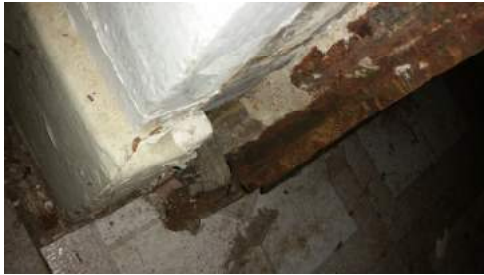
Duct Insulation, 1st & 2nd Floor & Basement
