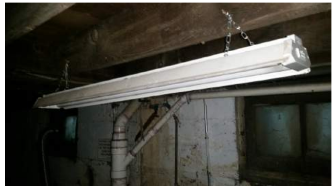
Ballasts, Fluorescent light tubes, 4ft or less, Room 12
