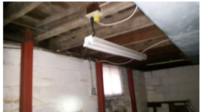
Ballasts, Fluorescent Light Tubes, 4ft or less, Room 11
