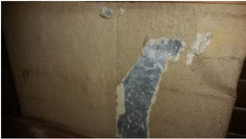
Duct Insulation, 1st Floor, 3 Duct Runs
