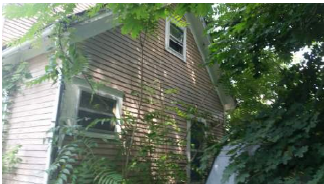
Back of house/property
