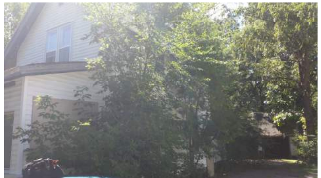
Side #2 of house/property
