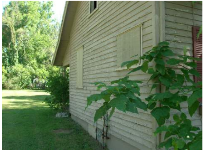
Side #1 of house/property
