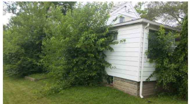
Side #2 of house/property
