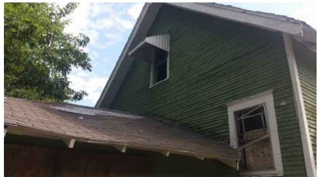
Side #2 of house/property
