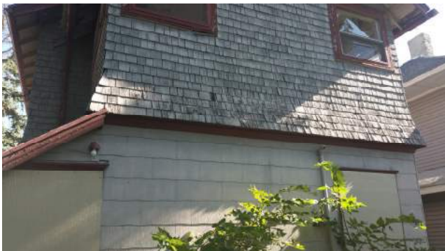
Back of house/property
