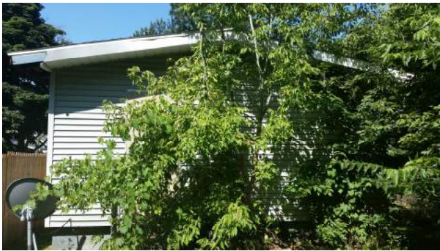
Back of house/property
