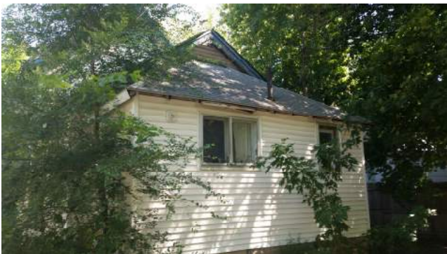
Back of house/property
