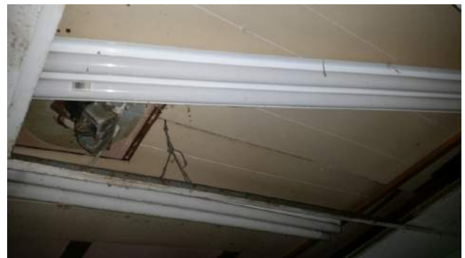
Ballasts, Fluorescent light tubes, 4ft or less, Room 2
