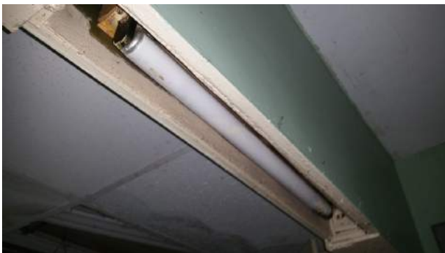
Ballasts, Fluorescent light tubes, 4ft or less, Room 2
