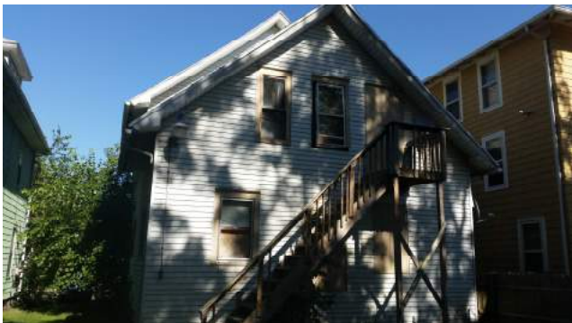
Back of house/property
