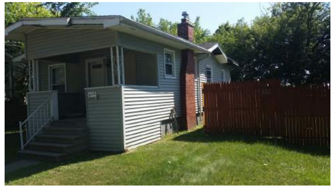
Side #2 of house/property
