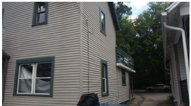
Side #2 of house/property
