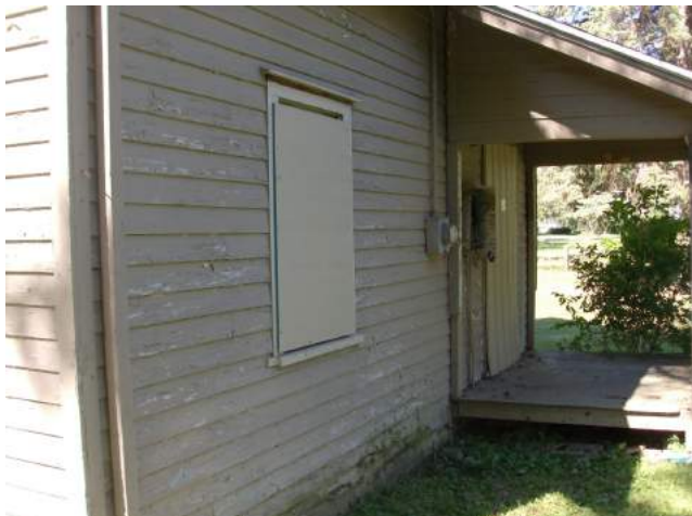
Back of house/property
