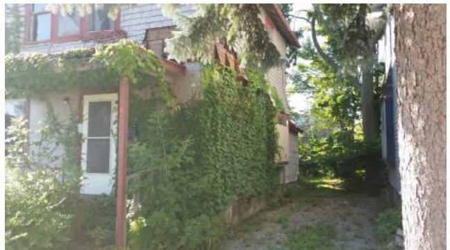
Side #2 of house/property
