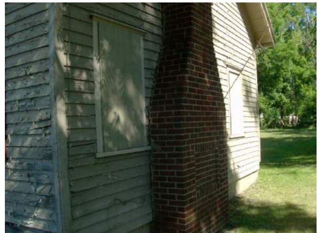
Side #2 of house/property
