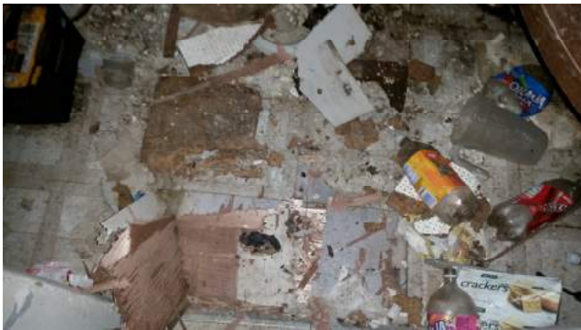
Floor Tile & Mastic, Room 7, 3rd
