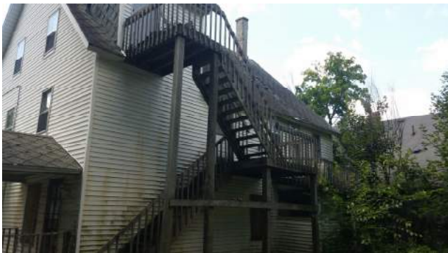
Back of house/property
