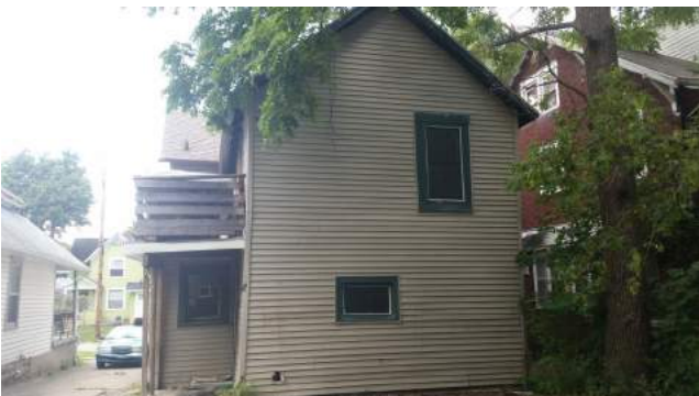
Back of house/property
