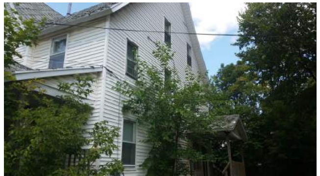
Side #2 of house/property
