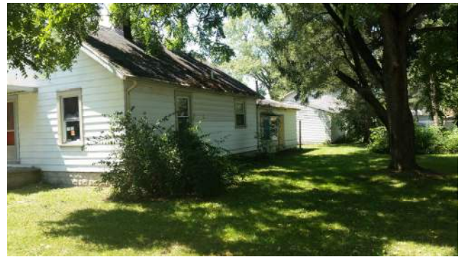
Side #2 of house/property
